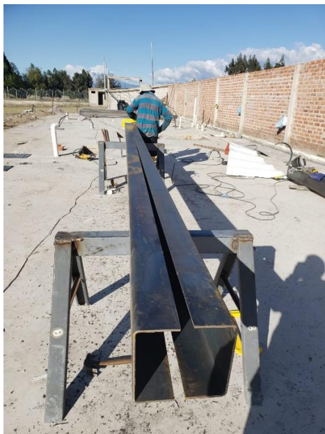
Columns being constructed for classroom building.
